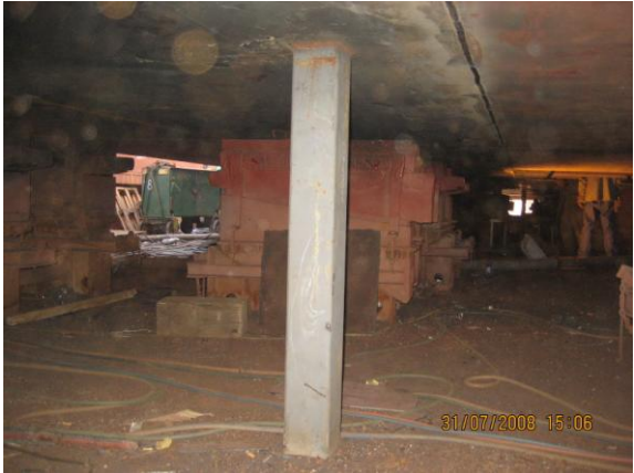
provisional supports in the repair area
