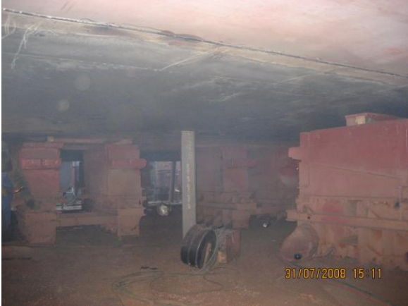
provisional supports in the repair area
