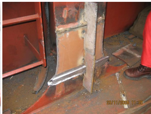
fitting a new section in-between the stays
