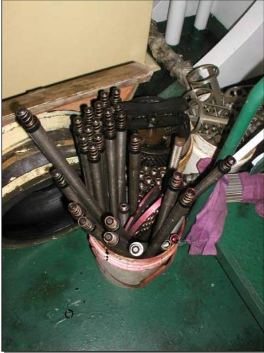
Improper storage of filter candles
